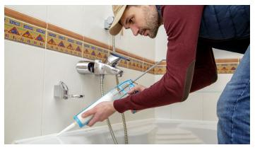
To prevent water from penetrating connections, corners and edges in the bathroom, the joints must be filled with silicone injected from a caulking gun. Thanks to its fungicidal content, the glossy sealant prevents mold growth in the warm and humid climate of wet areas. When using lowemission silicones with the EMICODE® seal, you can keep your exposure to possibly harmful substances as low as possible.
